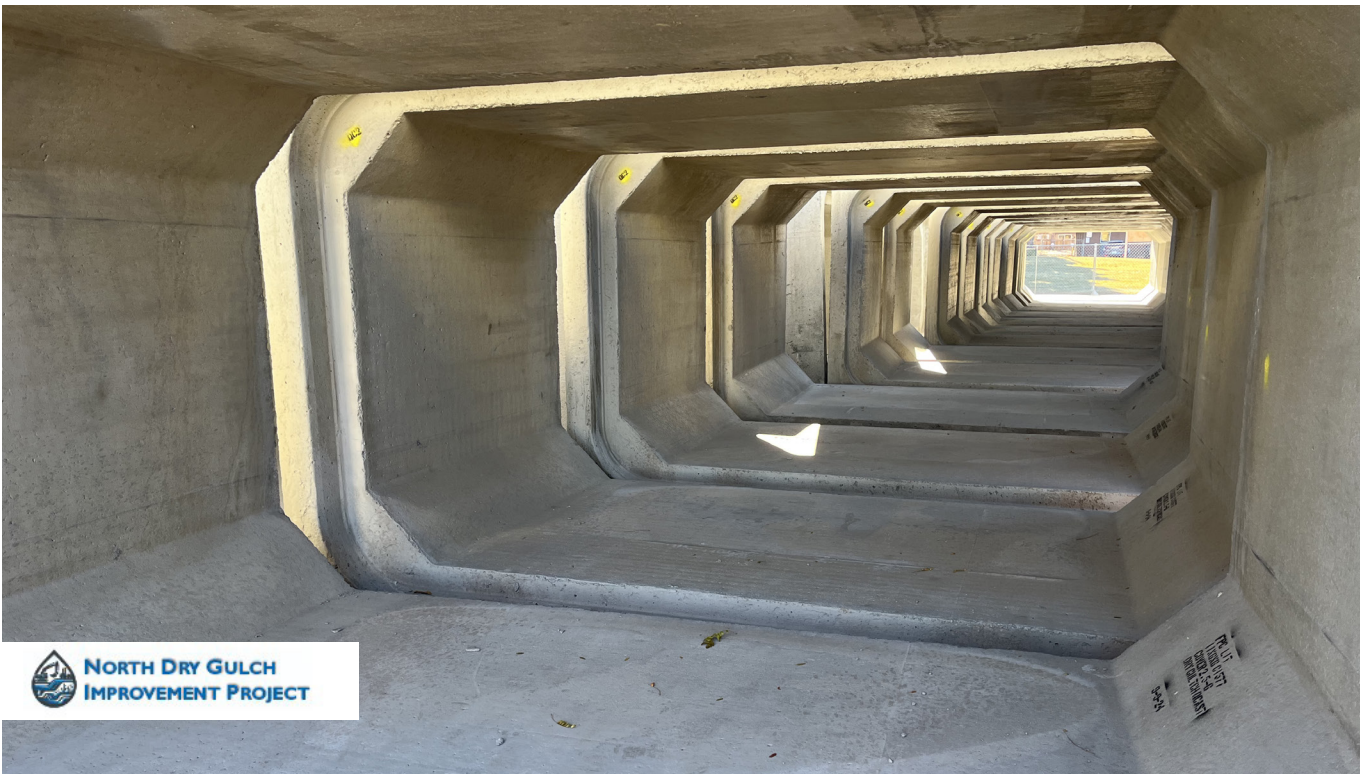
These large concrete conduits will help carry away stormwater runoff in the North Dry Gulch drainage, which will mitigate flooding in the West Colfax Avenue corridor.
