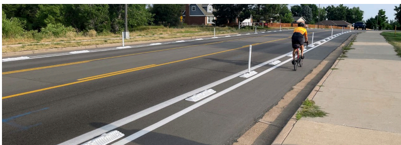
Figure E-4: Separated bike lanes constructed with plastic curbs and flexible delineator posts on Garrison St near Green Gables Park, 2024.
