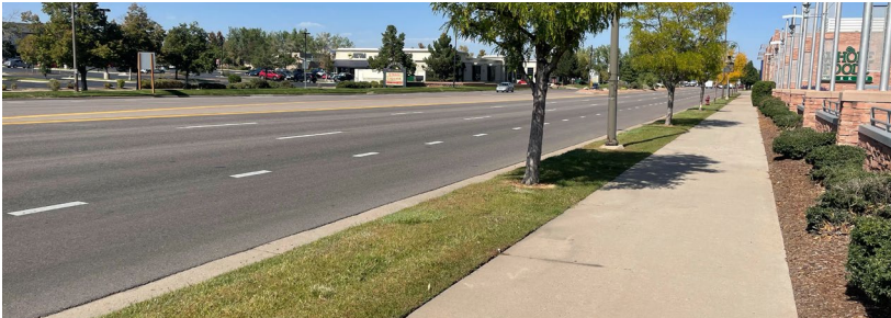
Figure E-8: A side path along Wadsworth Blvd near Virginia Ave, 2024.
